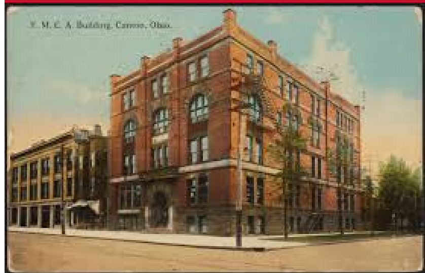
The original YMCA building located in Downtown Canton.
